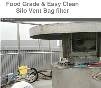
Silo Breathing Vent filter & Silo Top Level Sensor
