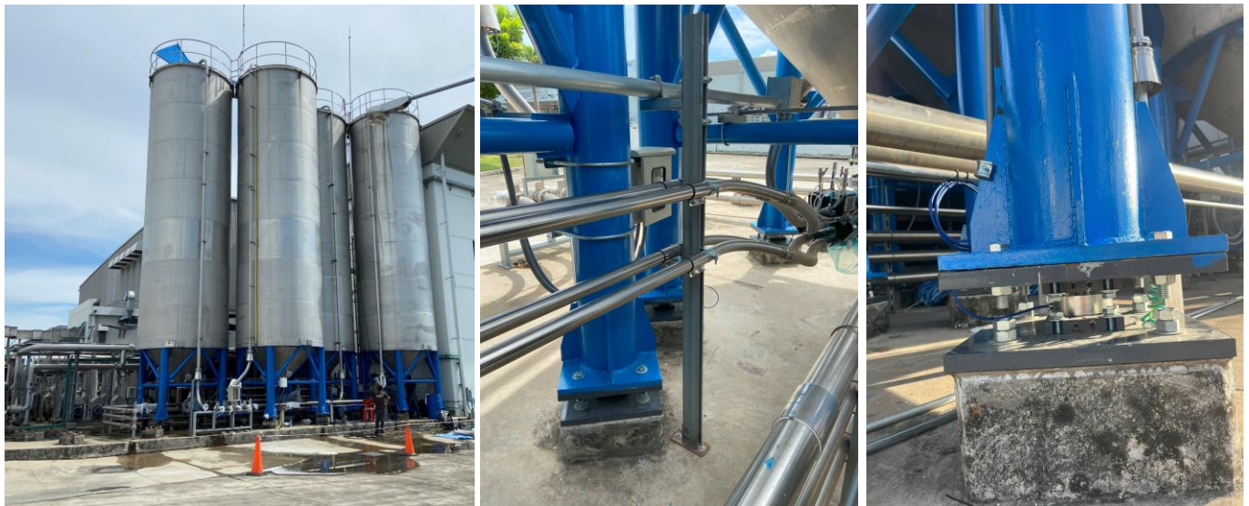
100 m 3 SUS304, PP, PE, PS & PET Storage Silos with Low Profile Pan Cake Load Cell Sets
