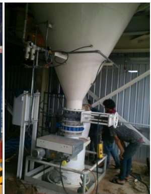
Silo Loading Bello with Over Filled Level Sensor
