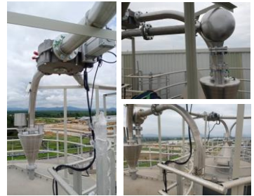
Feeding Pipe, Bends & Diverter Valve
