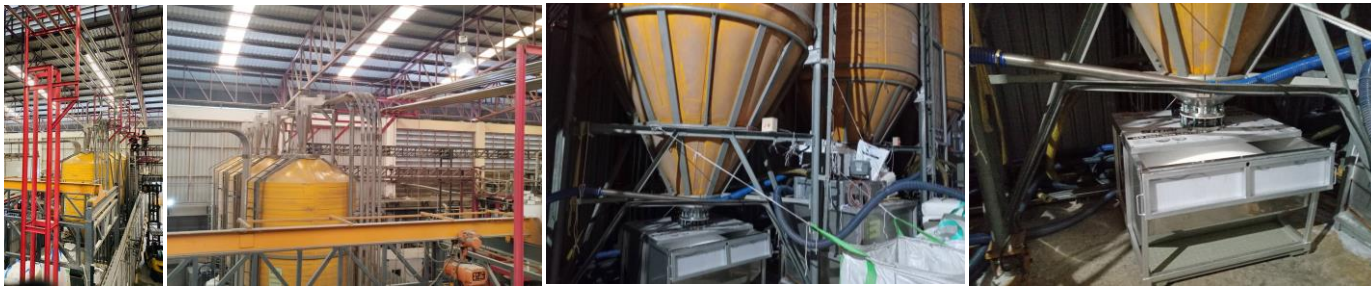
200 m 3 SUS304, PP Storage Silos with Shear Beam Silo Load Cell Sets
