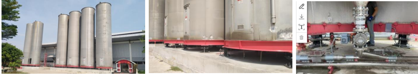
200 m 3 SUS304, PP Storage Silos with Shear Beam Silo Load Cell Sets
