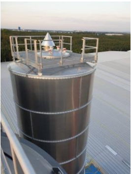
Silo Breathing Vent filter & Silo Top Level Sensor
