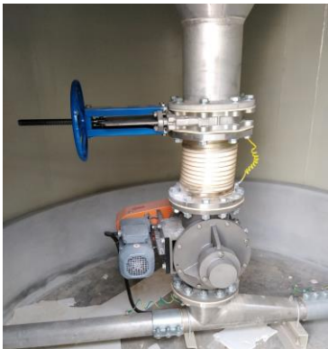
Slide Gate Valve, Flexible Connecting & Rotary Valve
