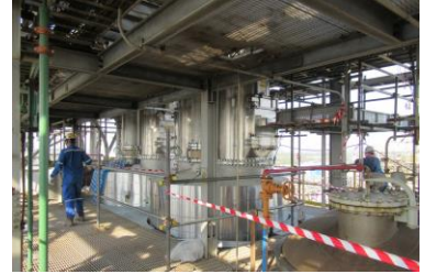
Feeding Pipe, Bends & Diverter Valve
