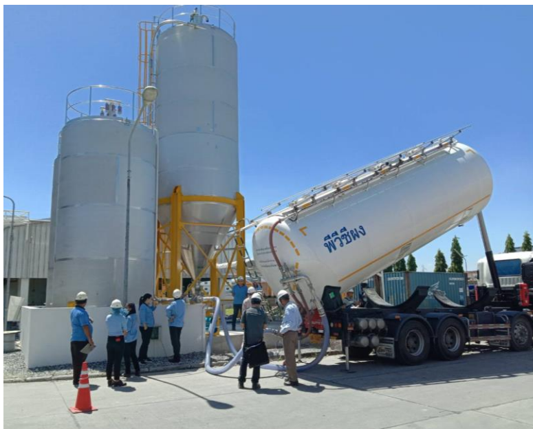
100 m3 PVC Storage Silo Load in by 16 Tons PVC Tank Car Designed Operation time in 60 minute
