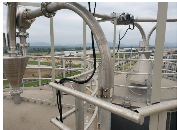
Silos Feeding Pipe & Valves Set
