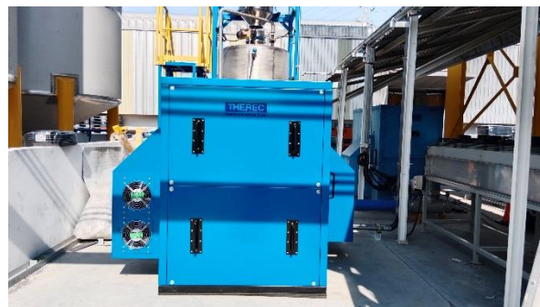
Roots Blower with Acoustic Enclosure
