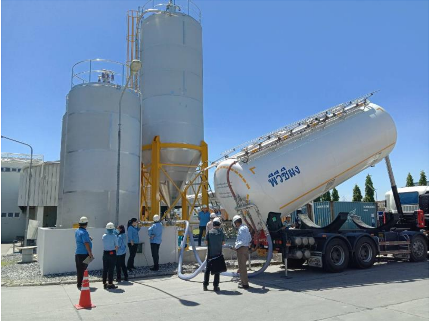
PVC Powder Silo loading & Weighting system / deliver from 16 tons bulk truck
