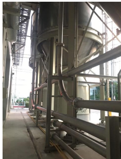
Silos loading system (PP&PE Pellet ) Fitesa CNC (CPPC group)
