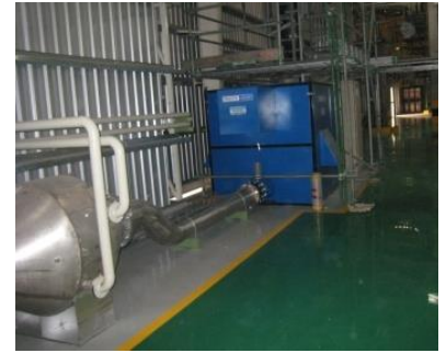
Roots blower package with air cooler set
