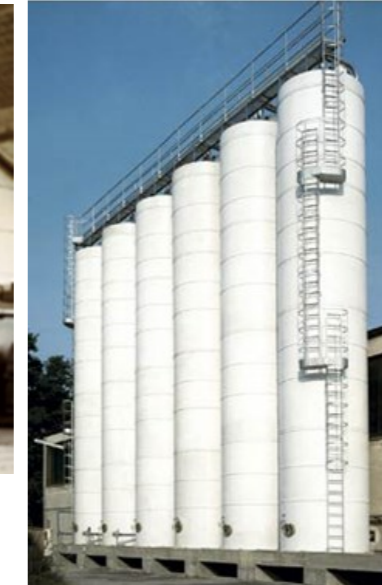
Silos in Vetroresina Reinforce Fiberglass
