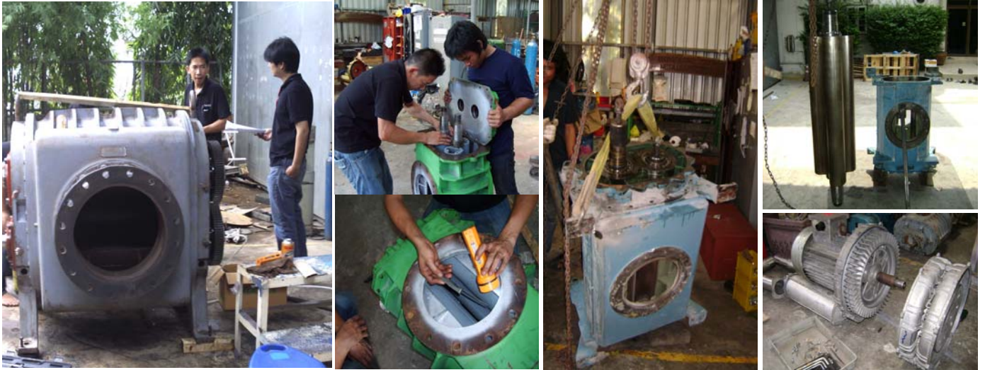
Service and Repair Work
