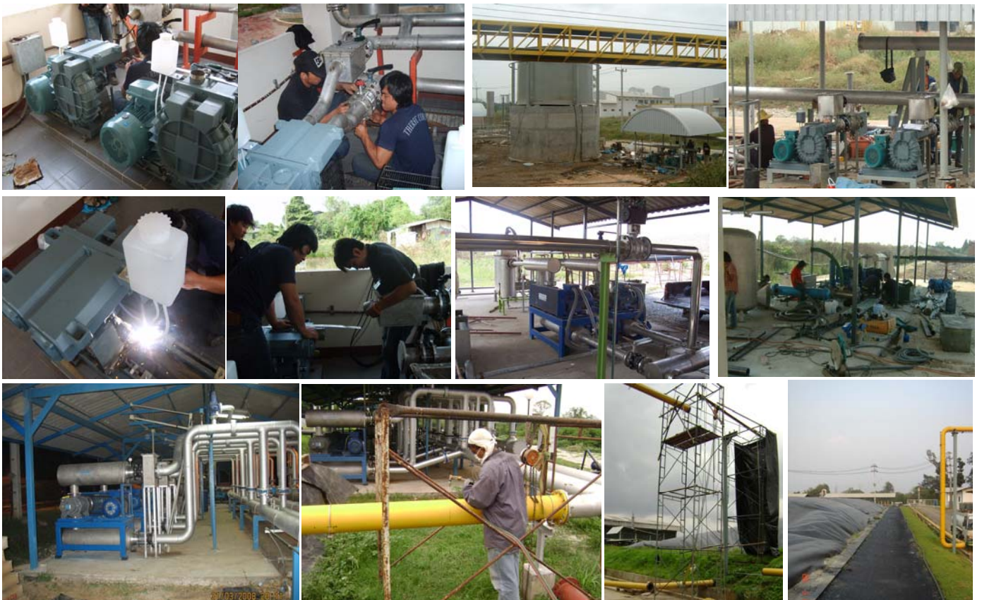
Installation Work Piping work
