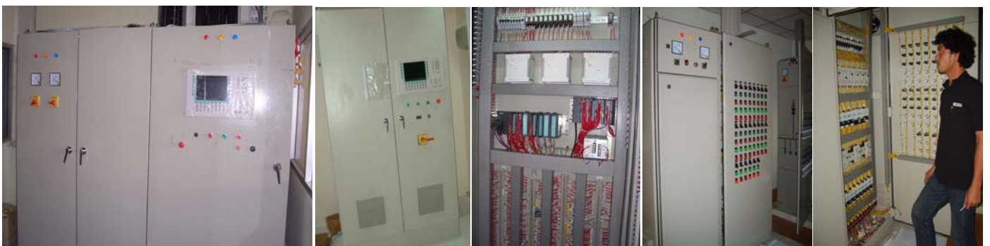
Electrical control work / PLC / SCADA system
